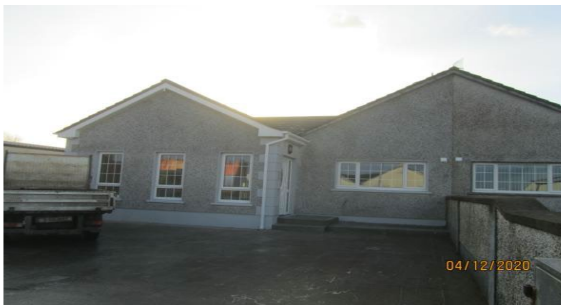
Bedroom extension to welfare unit
